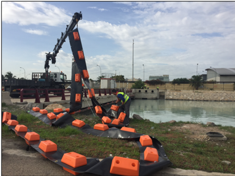
Photograph taken during installation of the barrier
