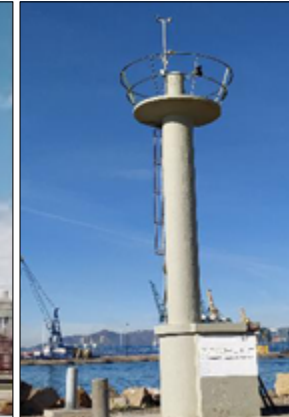
Weather Station Beacon at Levante Quay, Sagunto
