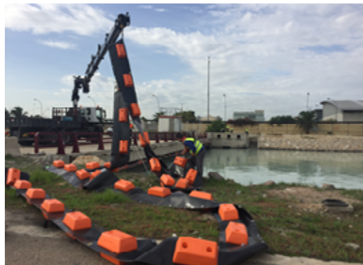
Photograph taken during the installation of the barrier.
