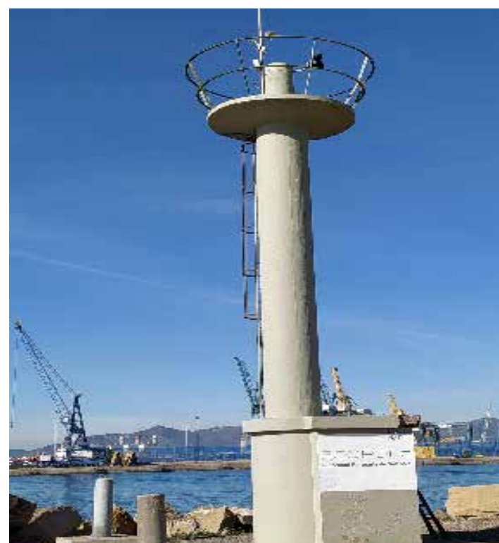
Weather Station Beacon Muelle de Levante Sagunto
